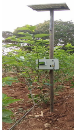
The Transmitter module installed in the field
